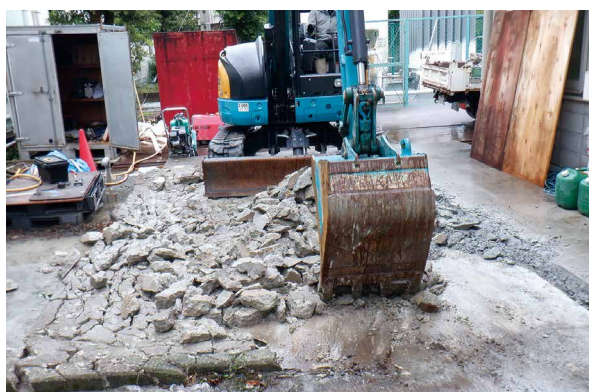
Takasago Plant low-concentration PCB waste treatment work under way
