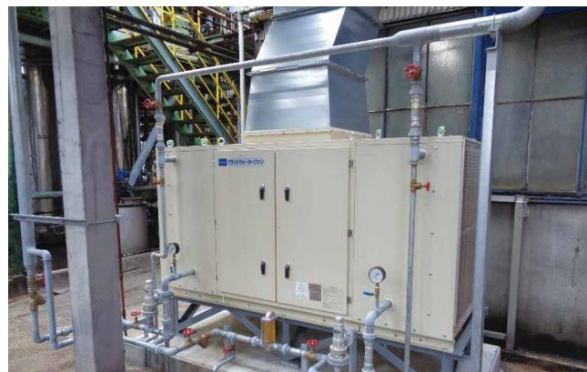
Main unit of heat exchanger-type cool air supply equipment
