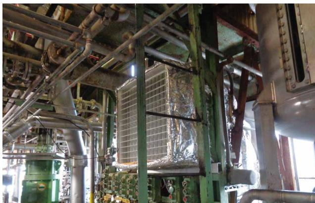
Outlet vent for heat exchanger-type cool air supply equipment
